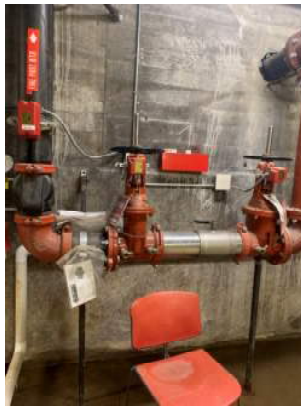
Existing Sprinkler Service Valves
