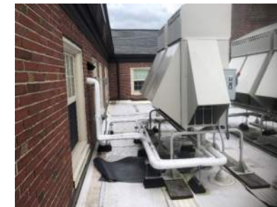
VRF Heat Pump Units (Typical Indoor Units @ Left & Outdoor Units @ Center & Right)
