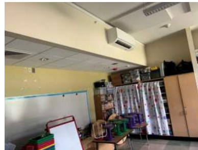
VRF Heat Pump Units (Typical Indoor Units @ Left & Outdoor Units @ Center & Right)
