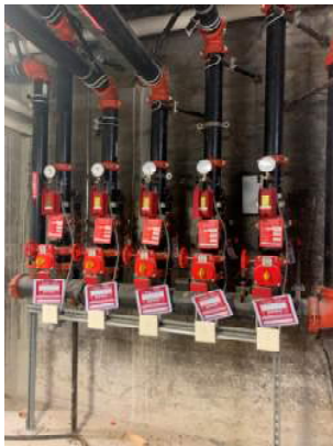
Existing Sprinkler Zone Control Valves
