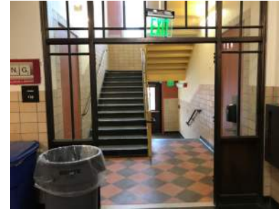
Stair Demo & Infill
