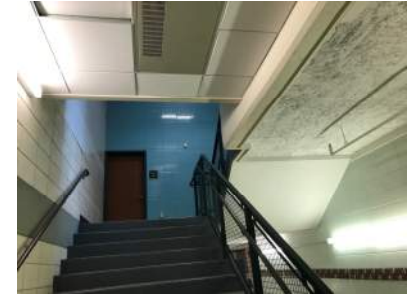
Stair Demo & Infill
