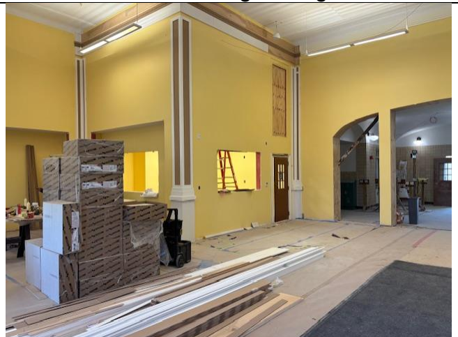
Installing Millwork in the Library
