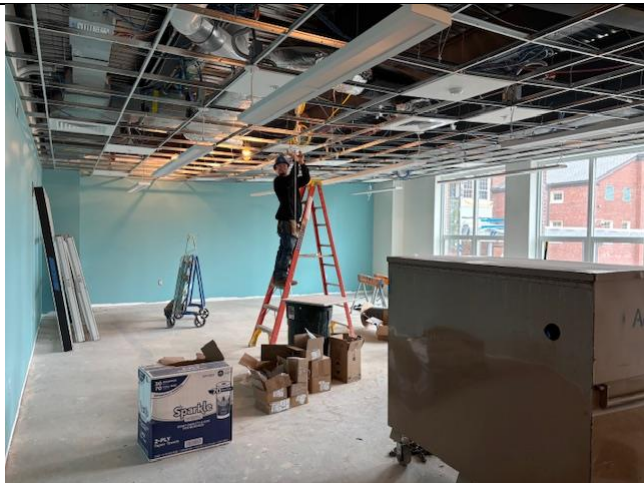
Installing FA Devices on the 1st Floor of the South Addition
