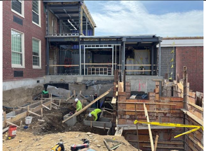
Formwork for Remaining Foundation Walls at the North Addition
