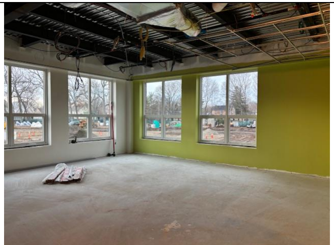
Painting begins at the First Floor of the South Addition
