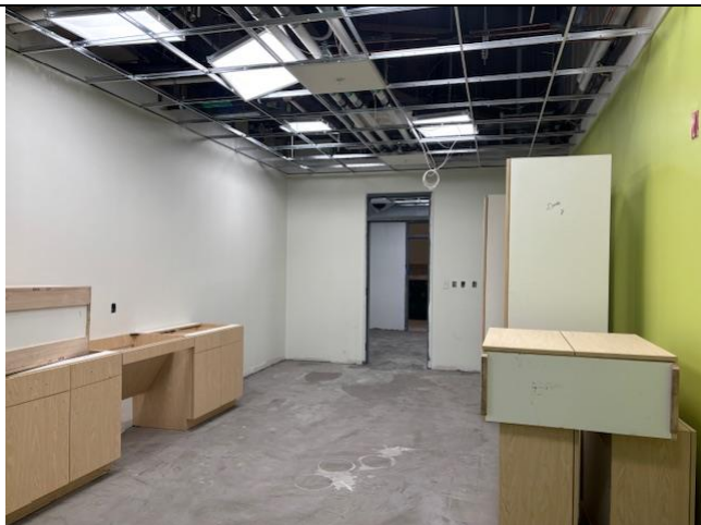
Installation of Cabinets Begins at the Staff Lunch Room
