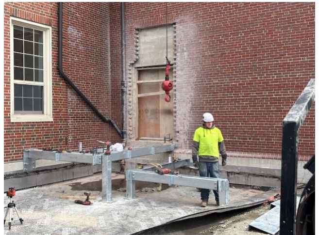
Steel Framing for the Accessible Ramp Begins
