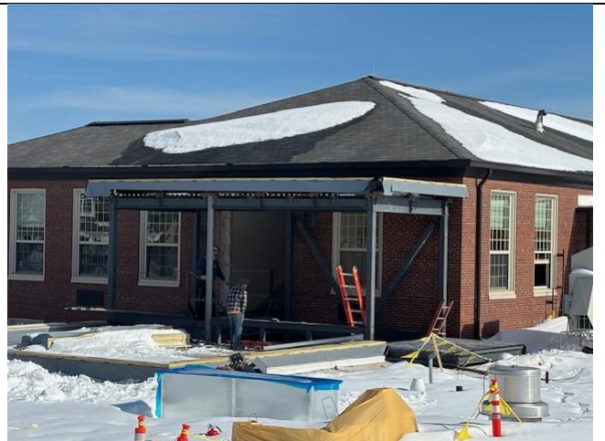
Finalized Steel Detailing at the North Addition
