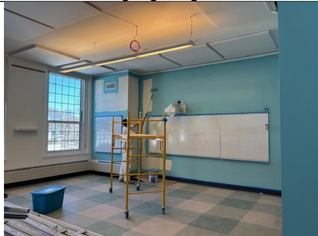
Painting Commences at the 2 nd Floor of the Existing Building
