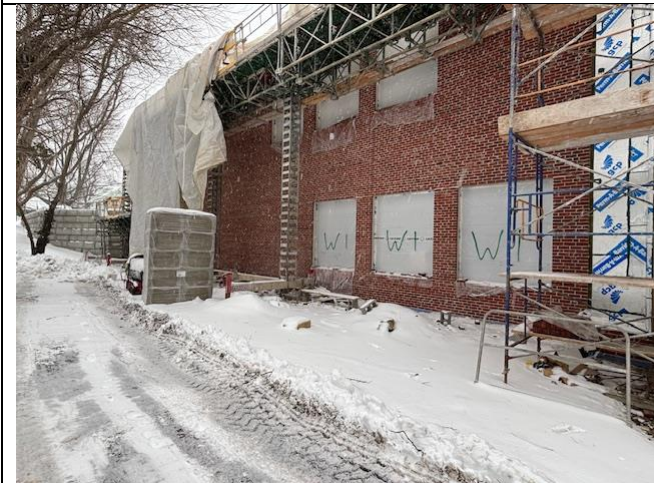
Brick Veneer is Ongoing along the West Elevation
