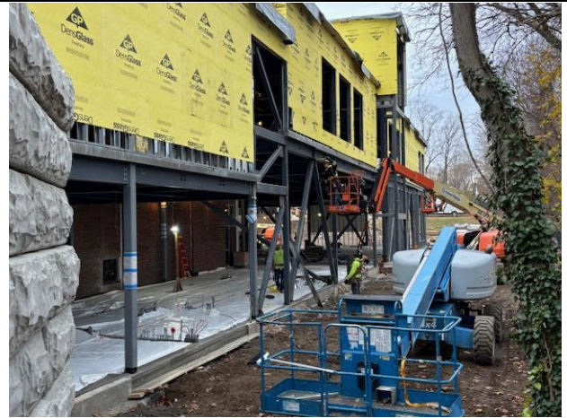
11/25/2025 – West Elevation Addition Sheathing installed
