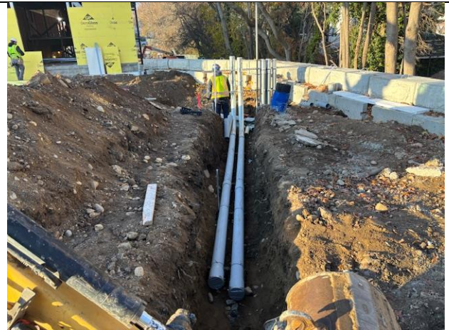
11/21/2025 – Duct Bank installation at Northern part of site
