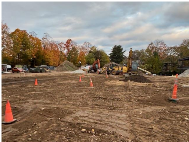
10/29/25 – Backfill and grading at Infiltration System 1 (Southern side)
