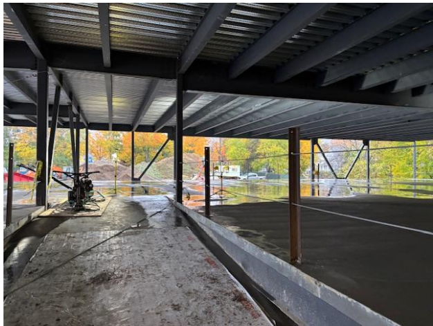
10/30/2025 – Completed Level 1 concrete placement
