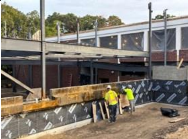
09/30/2025 - Sheet Membrane Waterproofing install at Foundation Wall along Lines A & 2.8
