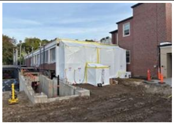
09/30/2025 - ACM Abatement Enclosure at Wall along Line XO
