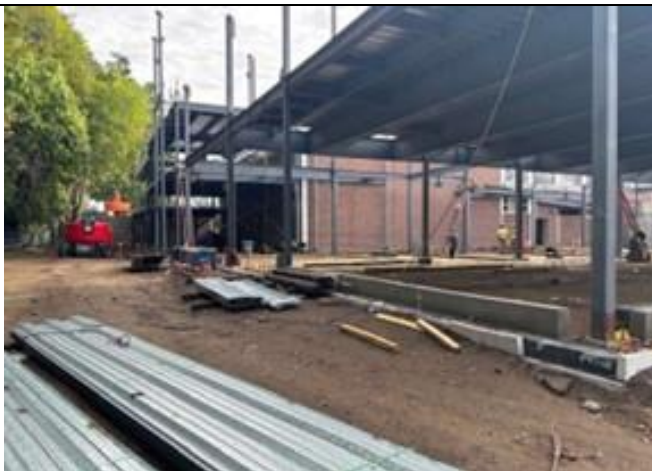
09/26/2025 - Detailing First Floor Sequence 1 Steel
