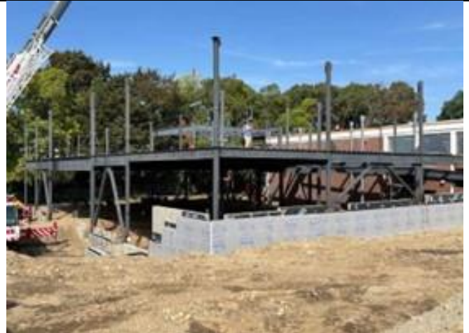
09/30/2025 - Sequence 1 Steel Erection and Detailing
