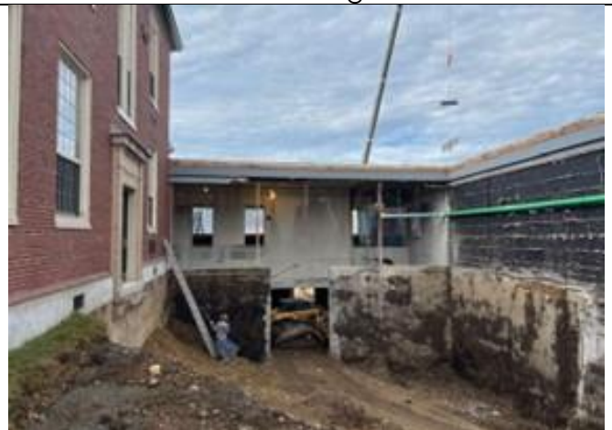
09/26/2025 - Loading Debris Out of the Building at the North Side
