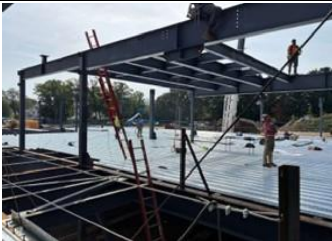
09/30/2025 - Sequence 1 Erecting 2nd Floor (Roof) Steel
